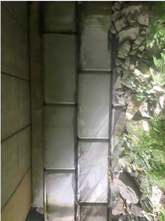
Left Bank Abutment when facing downstream
