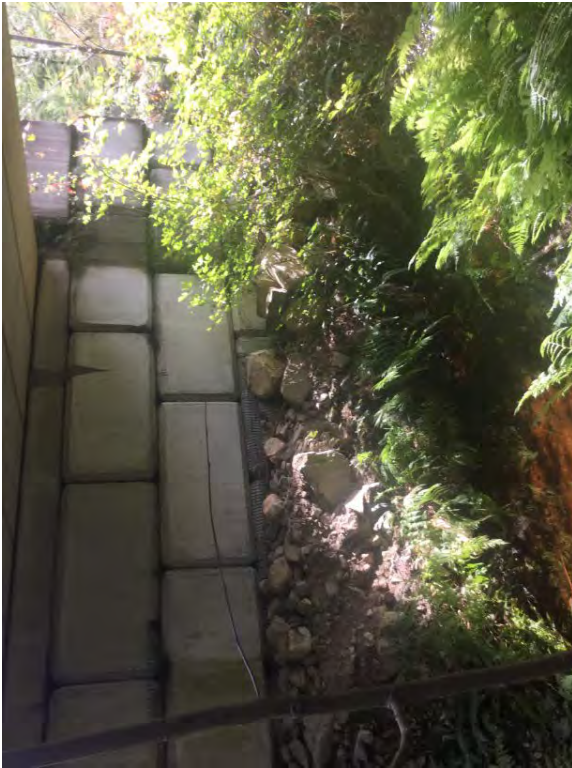
Right Bank Abutment when facing downstream
